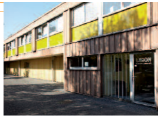
Head office and production site in France (Somain)
